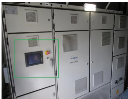
Armario ground, señalado en verde el panel de control Ground cabinet with the control panel outlined in green
